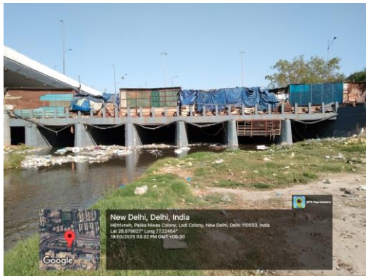
Inlet of the covered drain
