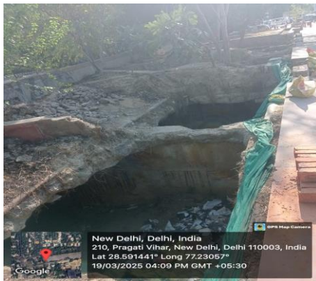
Inlet of the covered drain
