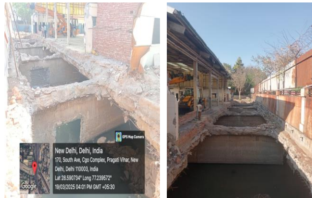
Outlet of the covered drain
