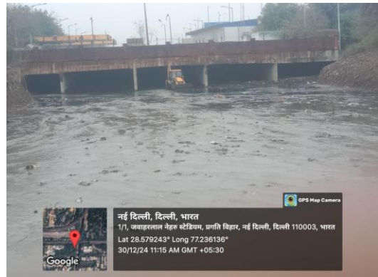
Outlet of the covered drain
